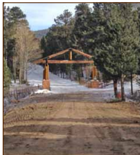
The main entrance to Land O'Peaks during and after the road repair process.
